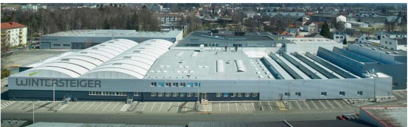
Headquarters located in Ried im Innkreis, Upper Austria
